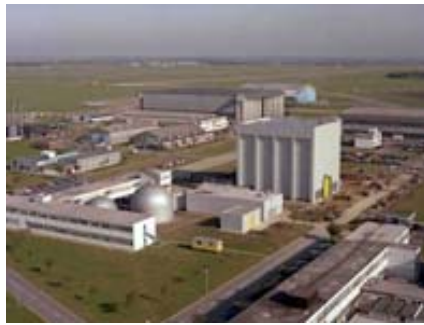
Bedford Enclave Showing the Newly-Completed Large Motion System Building, 1982 (B6088C)
