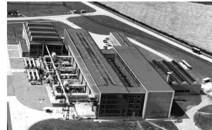
Exterior view of 3x4 (HSST) tunnel building, 1961 (neg C6568)
