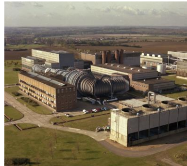
The 8x8 tunnel complex, a view taken in 1982 (neg B6087R)
