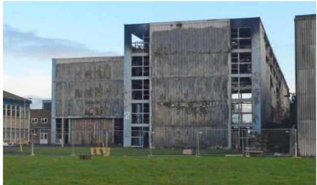
*HSST Buildings after the fire, Main Compressor Hall in front, with tunnel working section in building to the left (Image, from South, Barry Tomlinson P1120105)*
