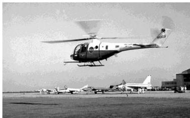
An unusual helicopter arrived one night by Hercules in October 1970: the Lockheed XH-51N (NASA 531) rigid rotor helicopter. The aircraft was on loan from NASA Langley to give the UK some experience with such a rotor prior to the first flight of the Westland Lynx - at that time a novel concept and an offering into an important Anglo-French collaboration defence procurement.
