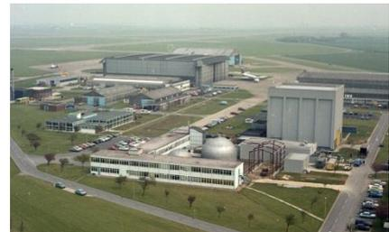
Most new buildings added to the main office area which became known as The Enclave, seen in the foreground of the picture, right (neg A4638, 1990), reflect the expansion of flight simulation as a research tool, from the two domes (1960s) to the huge box structure housing the Large Motion System (1980s). There were even more simulation-related buildings in the 1990s.
