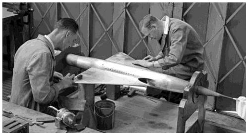
Models for the supersonic tunnels were generally made of high tensile steel, able to withstand the forces generated at high speeds (left, FD2 model being finished, *neg B4864-Bk1A, 1958*). Wooden models were appropriate for low speed testing in the 13x9.
