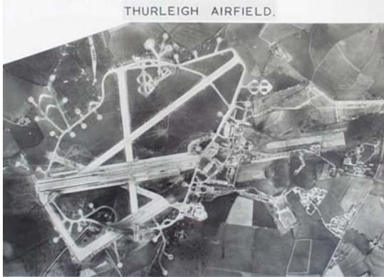
*Thurleigh airfield under construction, June 1952, showing the new alignment of the main runway*
