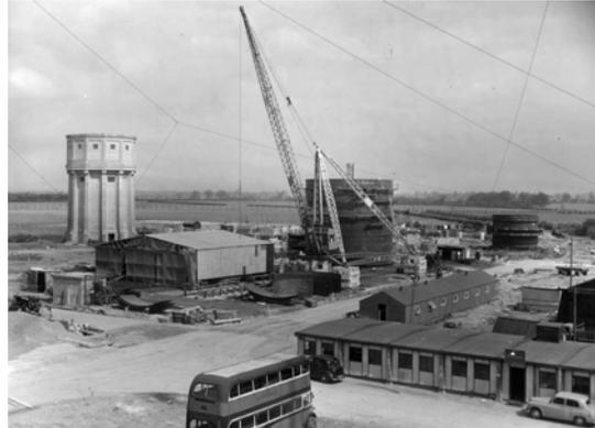
*Tunnel site, before move of water tower, April 1952, with steel sections of the 8x8 ft tunnel*
